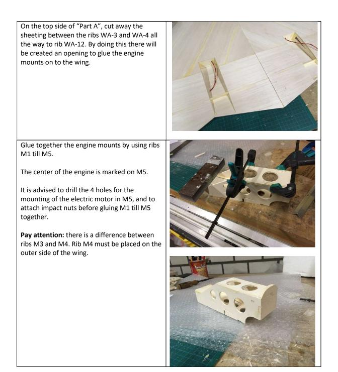
Attach the engine mounts in the created opening between ribs WA-3 and WA-4 with glue.
